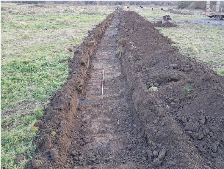
Plate 5: Trench 2 from northwest
