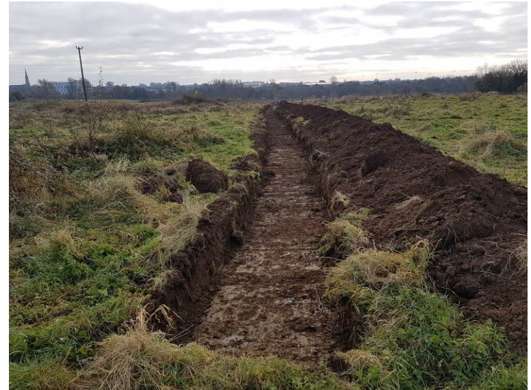
Plate 6: Trench 5 from northwest
